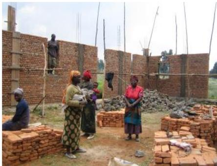
almost built and roofing sheets have been purchased. In the picture you can see steel rods built into the walls. They are there to protect against the earthquakes that can occur because the region is volcanic, and more steel rods will be added around the top of the walls.
